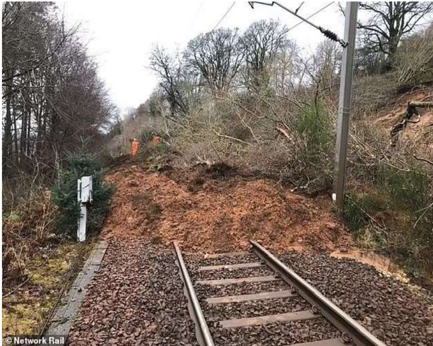
Fig – 7 – Landslide on the Railway line between Ardrossan and Largs in Scotland
